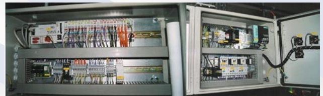
The switch cabinets are divided into a production part (right) and a control part (left), where the compact control system takes up a minimum of space.
